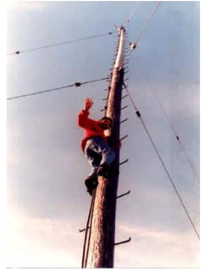
July 2000 - Maniitsoq Island (Greenland) Installing antenna on a very old tower !!!
